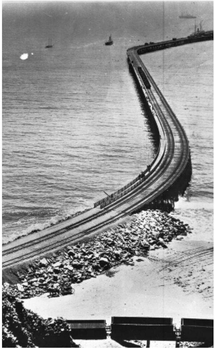
The Long Wharf, 1895. Credit: L.A. Water and Power
